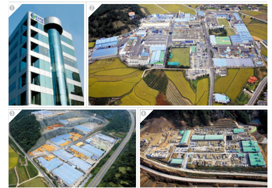
① Seoul Branch ② Head Office / Miryang 1 st Plant ③ Miryang 2 nd Plant ④ Hamyang Plant
